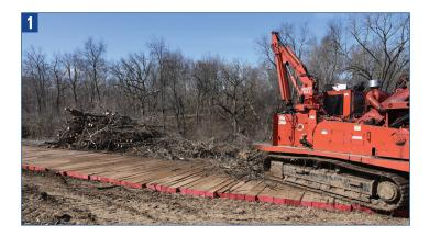
(that may look like a temporary road along the utility corridor) are often used to minimize compaction and soil disturbance and improve site safety. Using mats also helps speed up restoration efforts after the project is complete.
