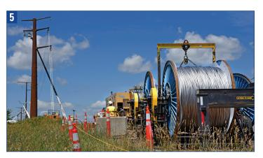
materials that that do not allow electricity to pass through them. Trucks, heavy equipment and sometimes helicopters, are used to string the lines. Other equipment, including bird diverters, spacers and devices to prevent the wires from galloping (moving up and down during icy, windy weather conditions) may also be installed.
